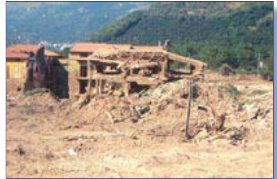
Above: The remains of a house after a landslide in Quindici, Italy. Source: www.land-man.net
