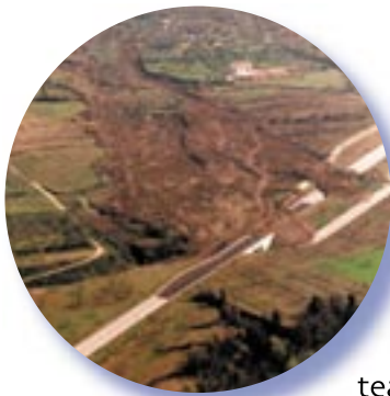
Left: Major road interrupted by a vast landslide movement.
